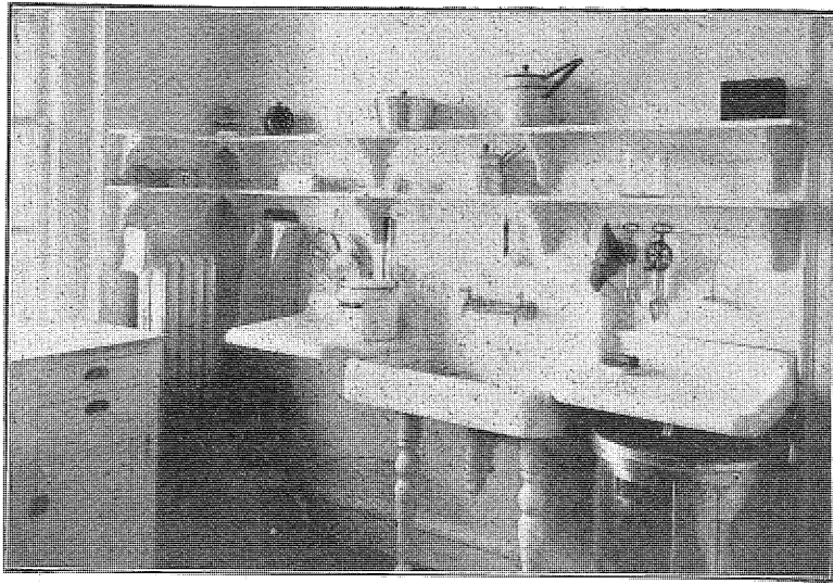
FIG. 7.—ARRANGEMENT OF EQUIPMENT AROUND SINK IN KITCHEN C
