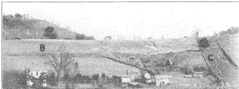
FIG. 8.—LANES OFTEN CAUSE EROSION
