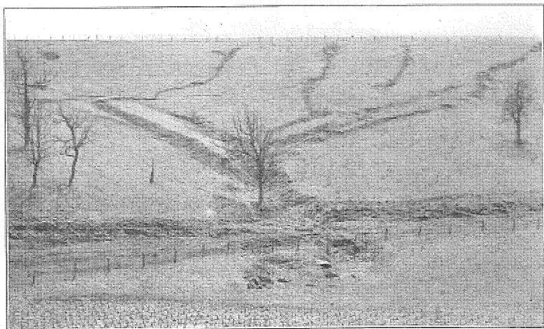
FIG. 1.—ABANDONED BECAUSE OF SEVERE EROSION
