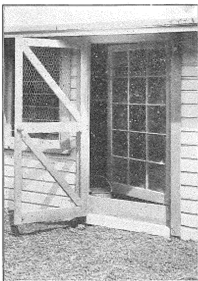
Figure 12.—Double doors are needed when it is desired to have a screen door. The inside door should be of glass and shorter than the other so it will swing over the litter.
